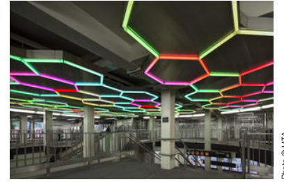
LED tubes, custom software, electrical hardware, aluminum, stainless steel
